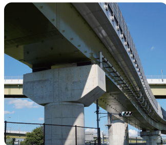
Highway Side Walls
